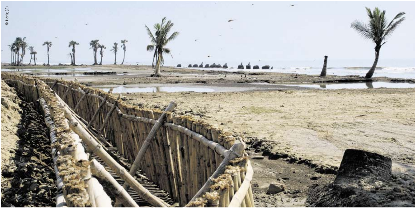
RESPECT FOR NATURE: Hurricane Aila ripped many trees from their roots. To protect themselves from further storms and floods, the people of Sibpur build dykes out of sand and clay, securing them with bamboo.
