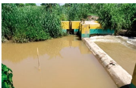
Irrigation weir at Ouanaminthe (Maribaroux). Source: Hauser
