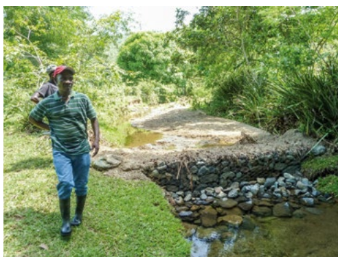
Erosion control with gabion walls and retaining walls and natural precautionary measures.
